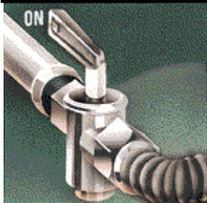
Appliance Gas Shutoff Valve
